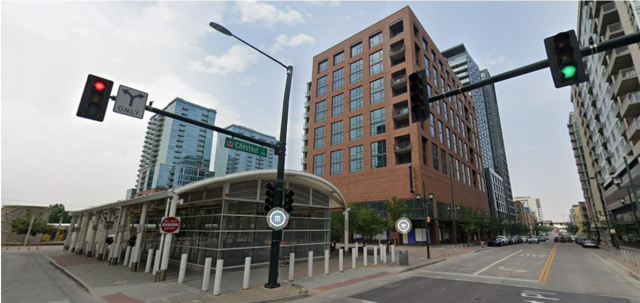
The entrance/exit to the underground Union Station bus terminal and the property beyond to the east of the subject property, looking northeast from the intersection of Chestnut Place and 17 th Street.
