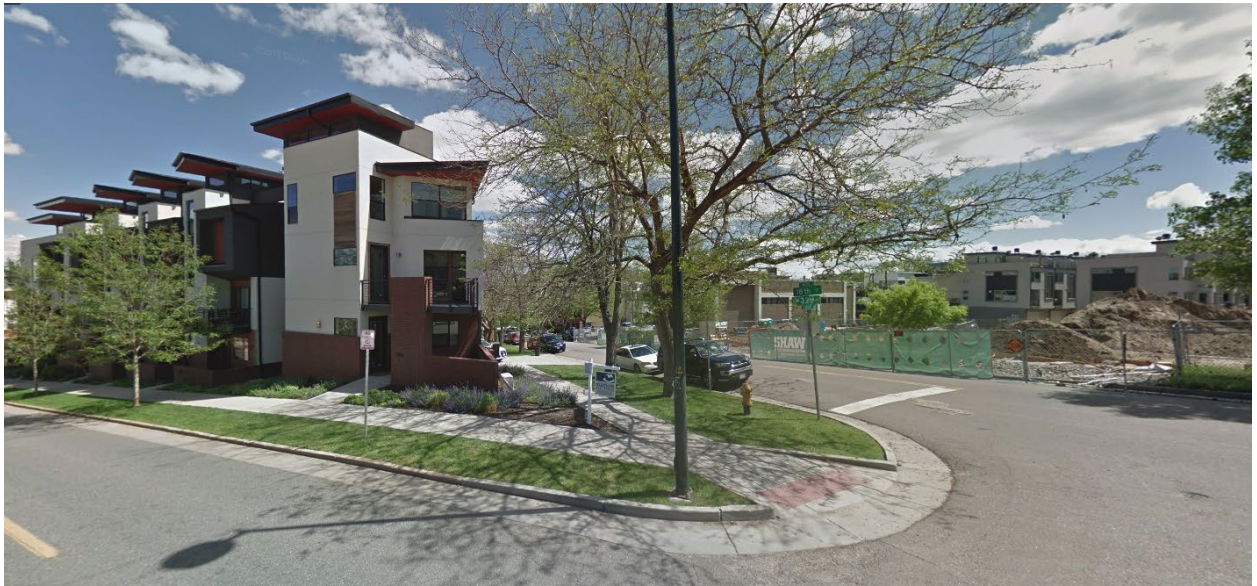
South – from 32 nd Avenue at 18 th Street
