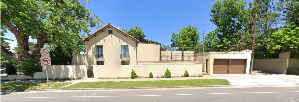
Subject Site – View of the subject property, looking north.
