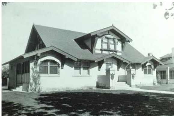
Early image of the 1906 Buchtel Bungalow, 2100 S. Columbine St. (Contributing to UPHD), designed by local architect Harlan Thomas. This was an early Modernist house and one of the first known houses built partially of concrete block in Denver. Source: DU Archives.
