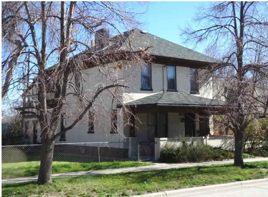
Image 18. The 1886 Clough House at 2525 E. Evans Ave. is the first documented house built in the University Park subdivision. Built by prominent Denver banker and cattleman John A. Clough, the residence has housed a prominent clergyman and DU faculty and students over the years. A caretaker for the large vacant acreage of University Park lived in the house beginning in 1886.
