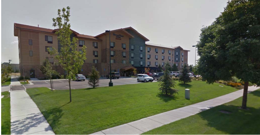
Subject site looking east
