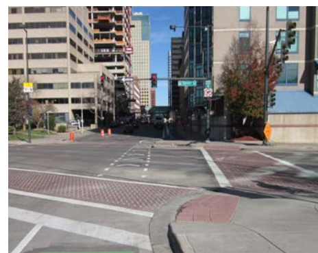
Example of a high-quality pedestrian crossing on Speer Boulevard
