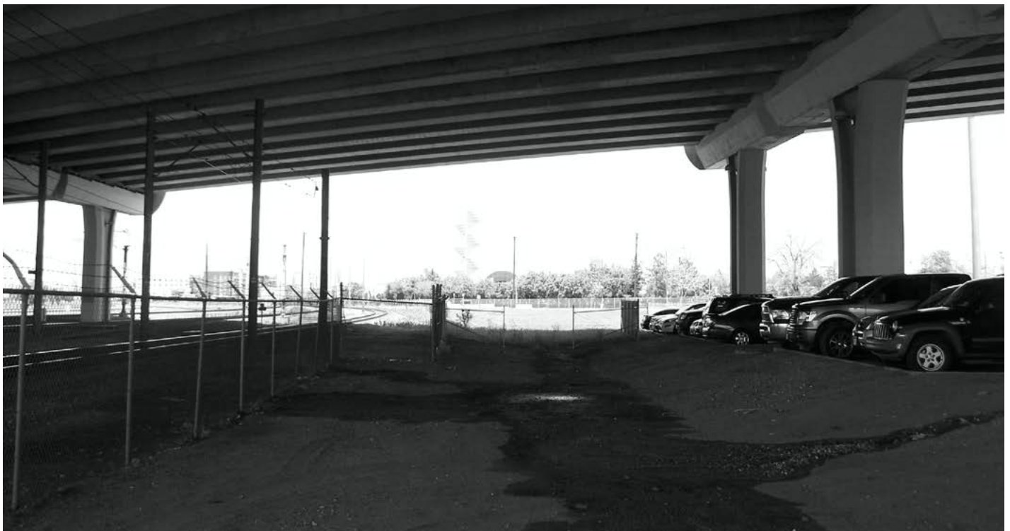
Existing conditions under the I-25 overpass.
