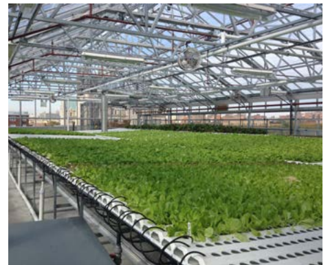
Rooftop greenhouse. Bronx, NY
