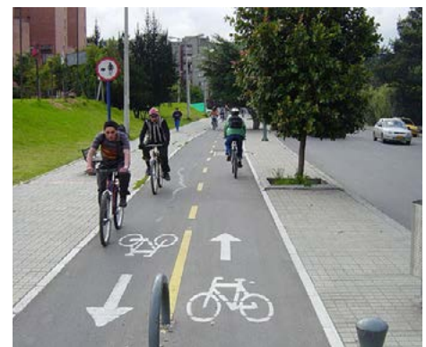
Protected two-way cycletrack
