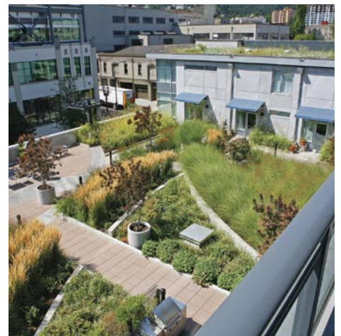
Green roof as usable outdoor space helps to reduce the heat island effect
