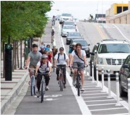
Buffered bike lane adjacent to vehicular lane
