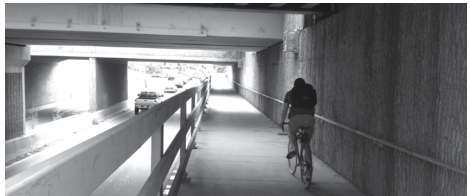
Existing condition along Mississippi Avenue underpass
