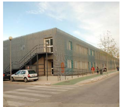
Retrofitted industrial building facade.
