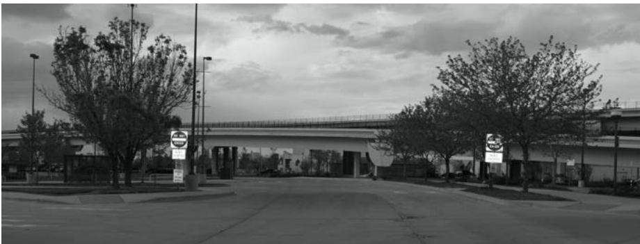
Existing I-25 and Broadway Station parking lot
