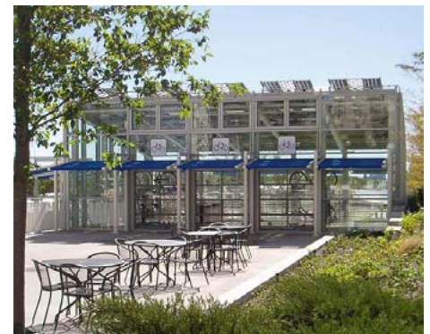
A bike parking facility includes secure bike storage.
