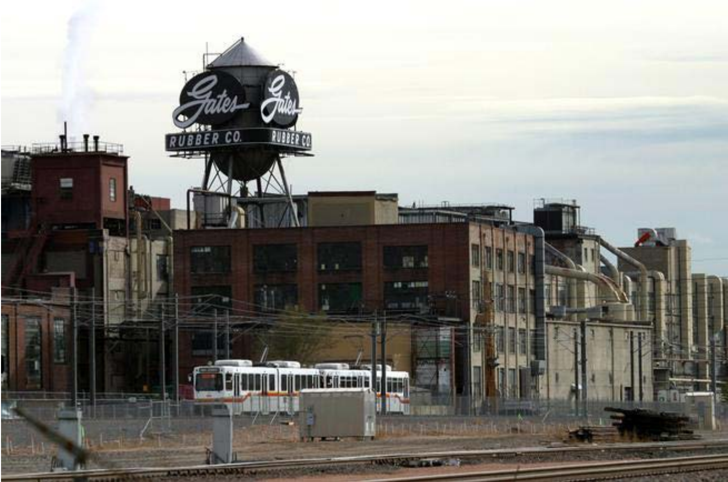
Gates Rubber Factory prior to demolition
