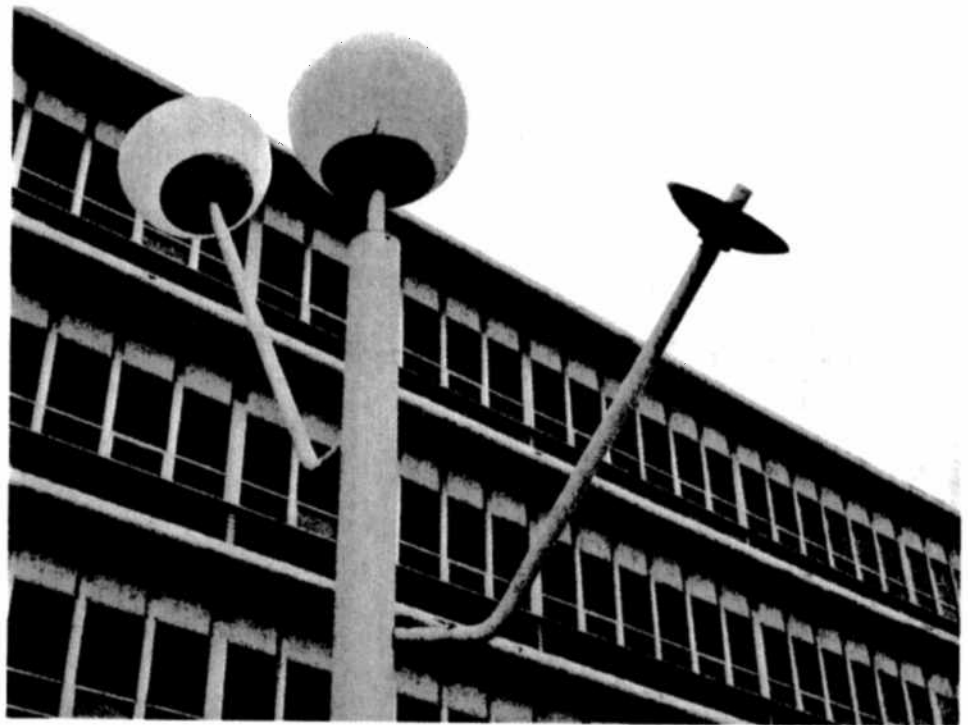
Outdoor light fixtures in the Study Area often were missing bulbs or other glass elements
