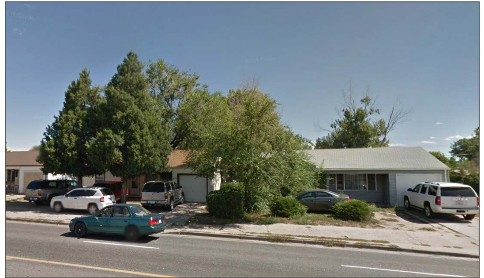
Existing attached sidewalk through south segment of project poses safety issues due to proximity to high volume roadway
