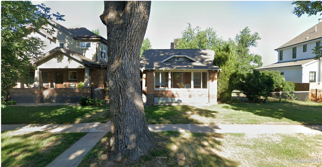
View of the properties to the east of the subject site, looking west from S Corona St.
