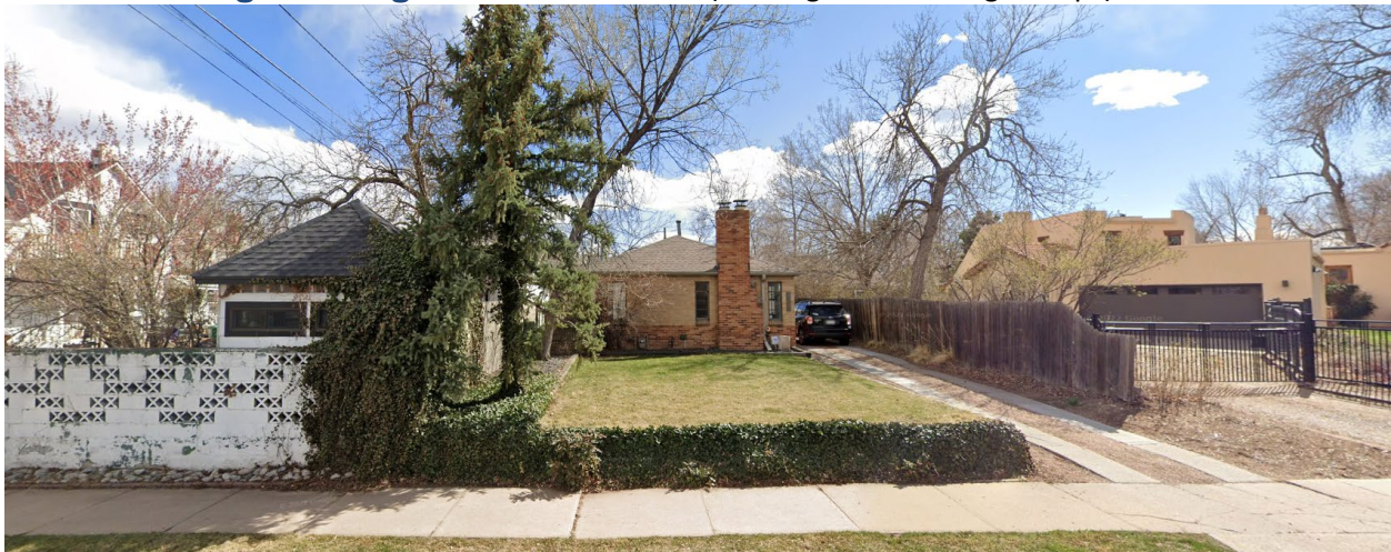
Subject Site - View of the subject property, looking south.
