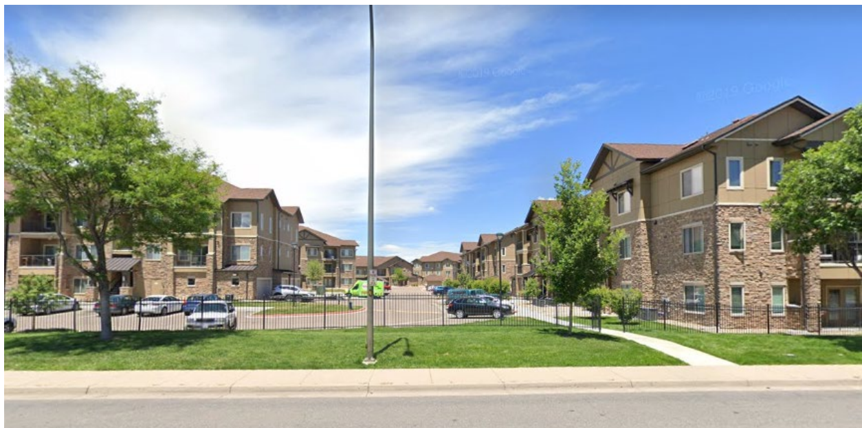
View of the property to the south looking north.
