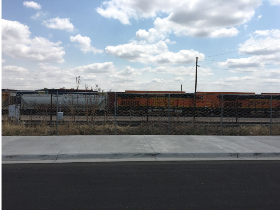
View of the freight rail tracks due east of the subject site, across Inca Street.
