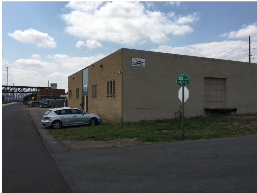
Industrial property located south of the subject site, across 42 nd Ave. The new pedestrian bridge for the 41 st & Fox station can be seen in the distance, one block away.
