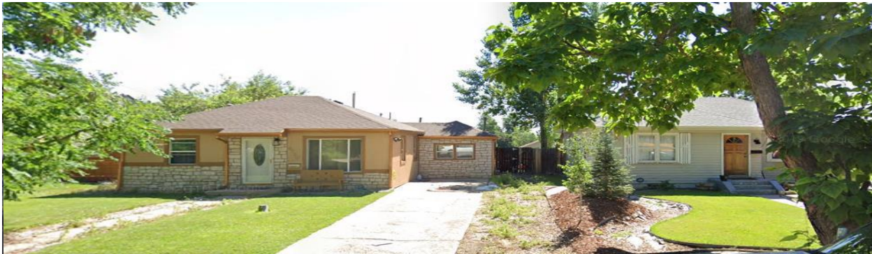
View of the 4722 and 4730 Clay properties, looking east.
