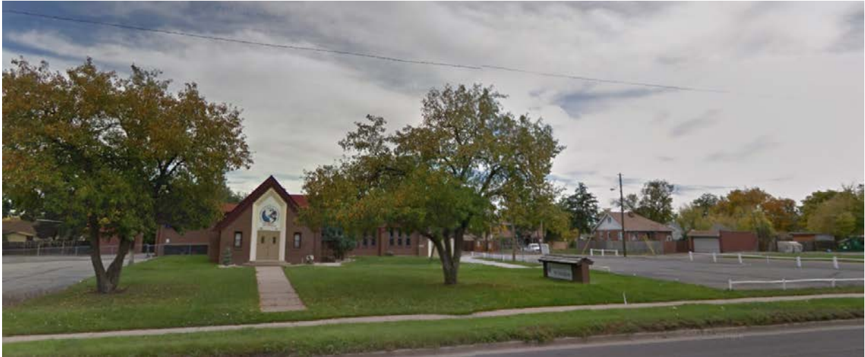
Site: 1 story Church
