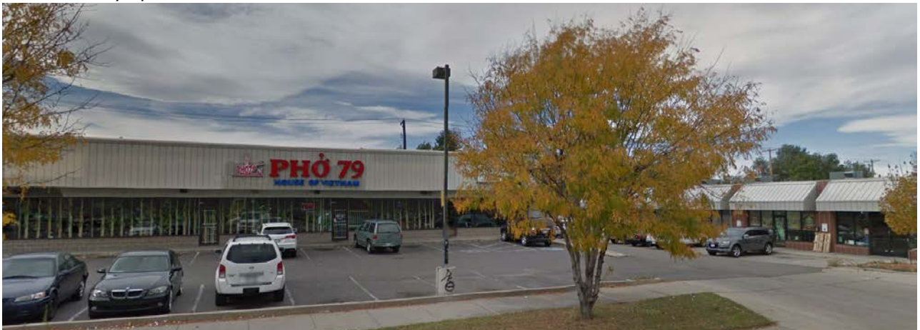
West: 1 story Commercial across Federal Blvd
