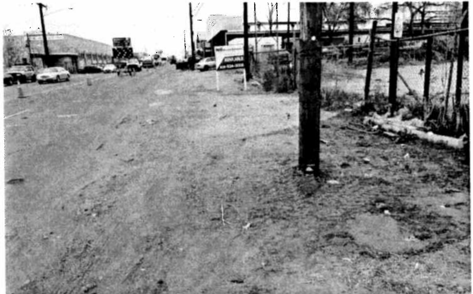
There was no curb, gutter, or sidewalks along Brighton Blvd adjacent to the Study Area
