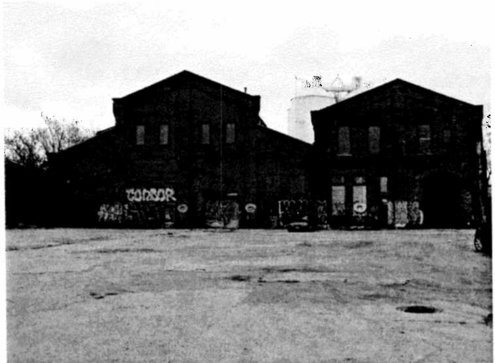
The warehouse structure sits vacant and unused
