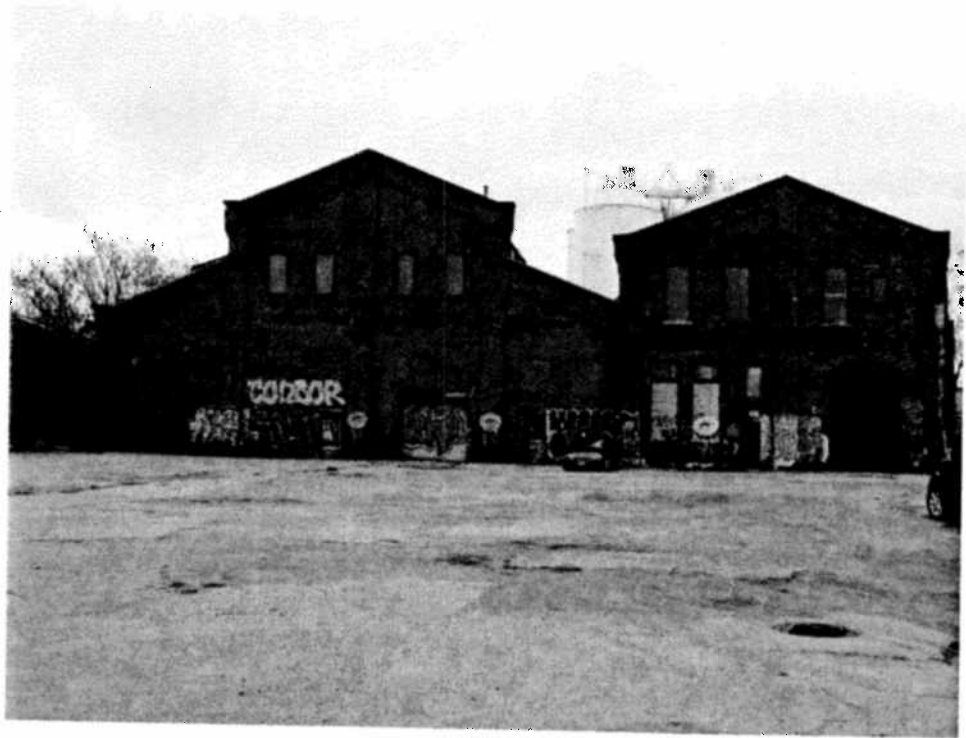
The overall structure had numerous boarded windows & doors, and graffiti proliferated throughout the exterior and interior
