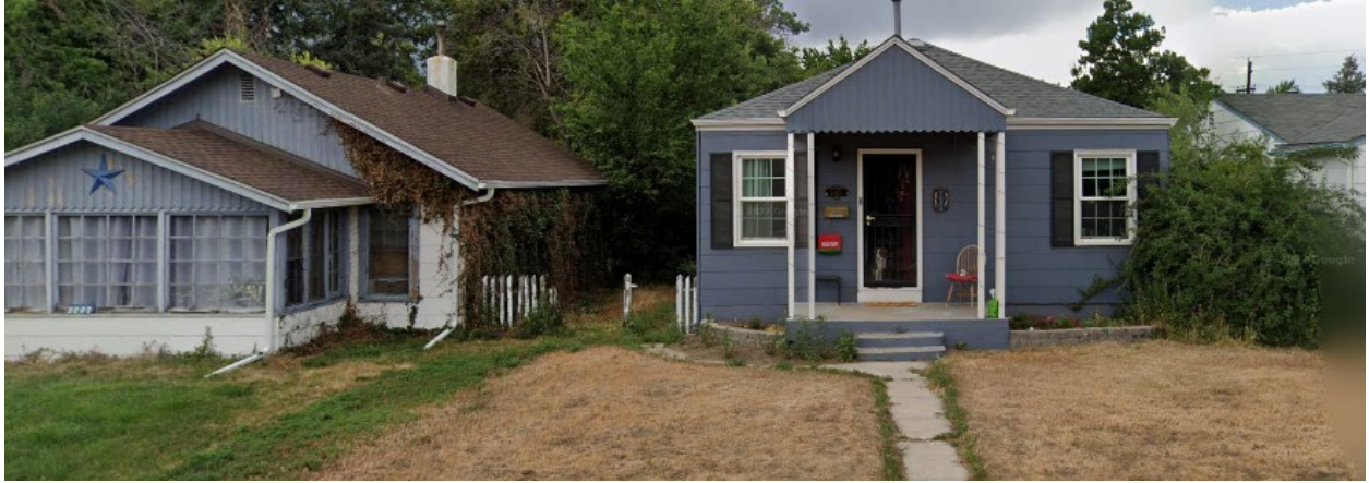
West - View of the properties to the west, directly across the street from site, looking west.
