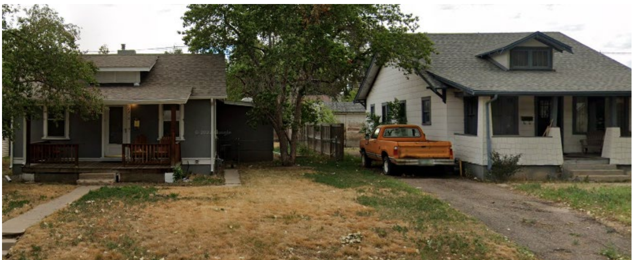
East - View of properties to the east, looking west (Gilpin Street)
