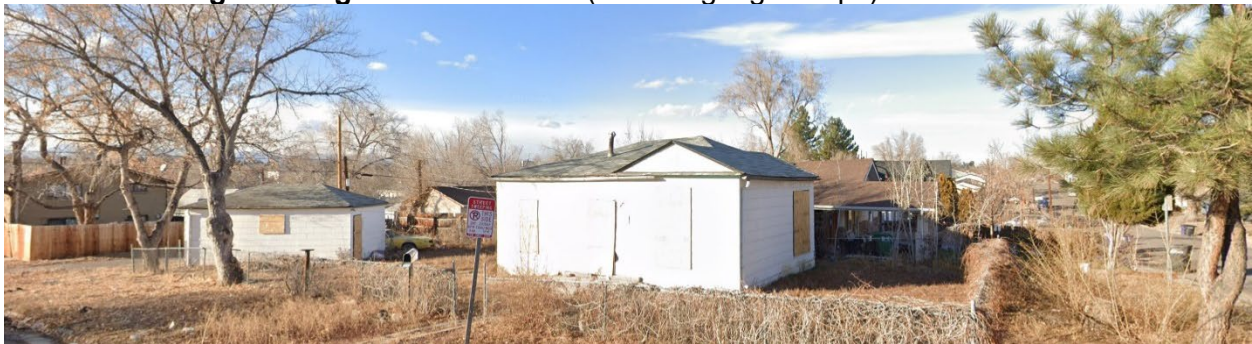
Site – Looking northwest at the corner of West 9 th Avenue and Meade Street
