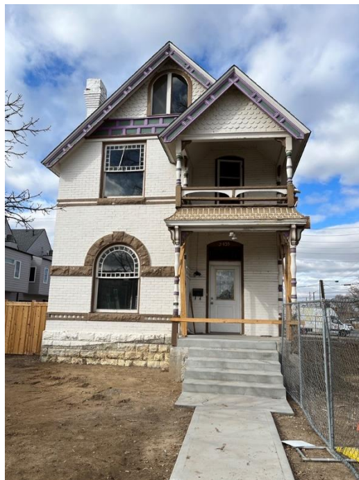
The Front (East) Façade of the Robinson House.
