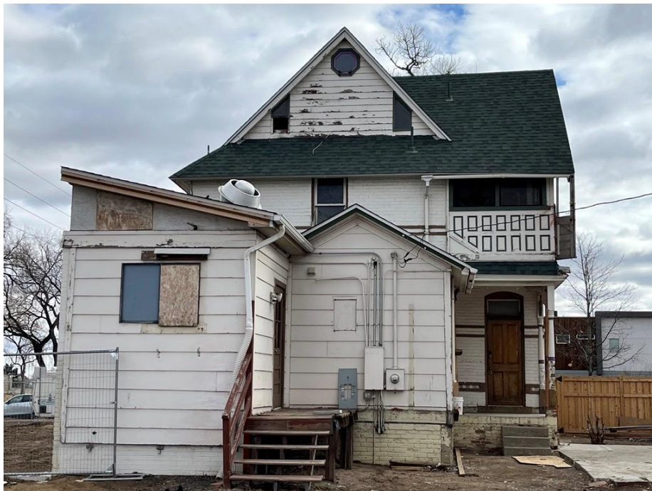
Robinson House, the west façade showing the original structure (top), 1913 kitchen addition (right), and 1980s addition (left).
