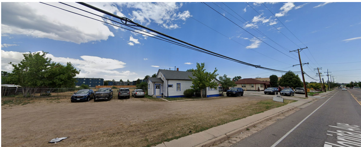
3237 West Florida Avenue - View of the subject property, looking northeast.
