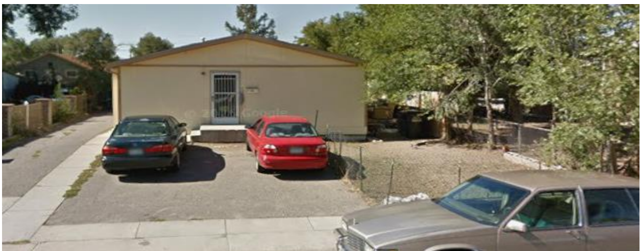
East - View of the property to the east, on Perry Street, looking west.
