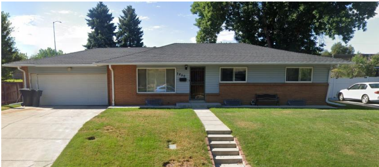
View of 3450 S Patton Way, looking south. (Source: Google Maps)
