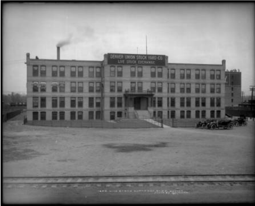
Figure B-1. 1908 photo of the 1898 Livestock Exchange structure showing the original facade, portico, and corner finials. 80
