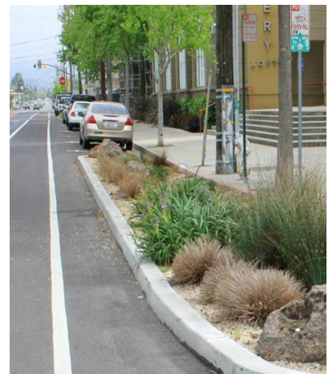
Bump-out Stormwater Planter
