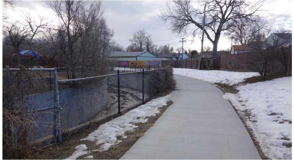
WEIR GULCH: EXISTING CONDITION
