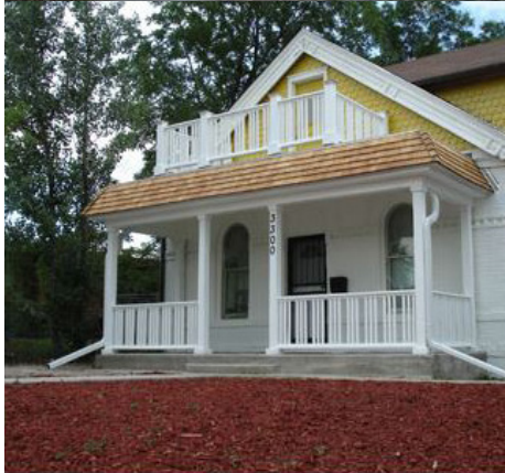
DURA Single Family Home Rehab Program Before and After
