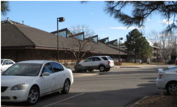
Office Building on subject site.
