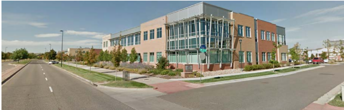
Image source: Google, image date: September 2011
