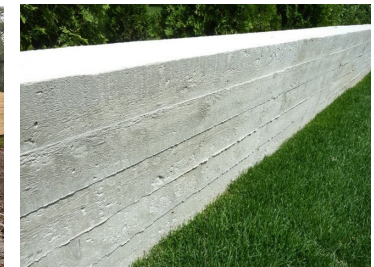
Board formed concrete retaining wall
