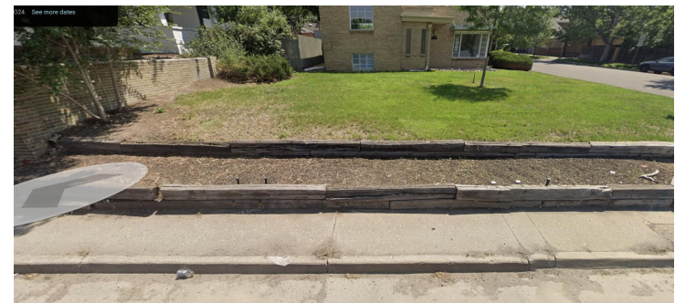
Existing retaining walls to be combined into one concrete retaining wall
