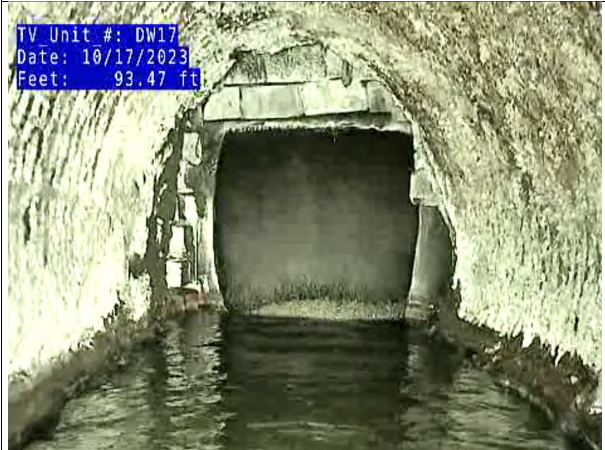
Graphic 2 - CCTV from segment 33854SAGM looking downstream at manhole 15666SAMH.
