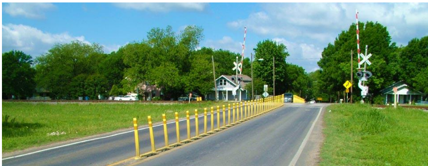
Two-gate with roadway channelization
