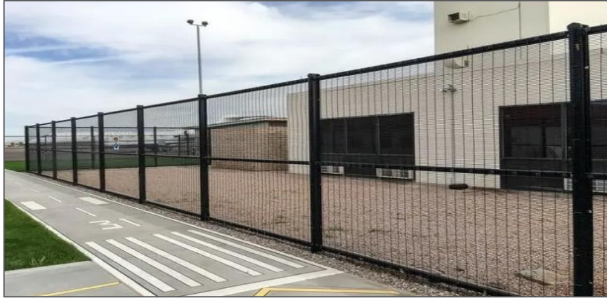
Anti-climb fencing to prevent trespassing
