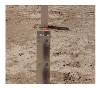
**Drilled Pier Mounting System**
