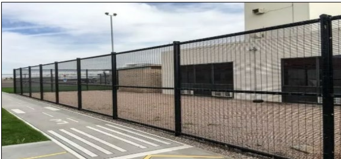
Photo 7-2. Example of Anti-Climb Fencing
