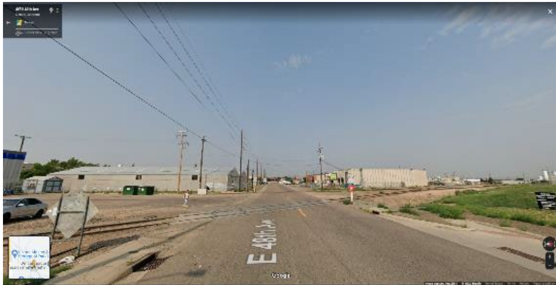
Photo C-7. East 48 th Avenue at Ash Street Crossing
