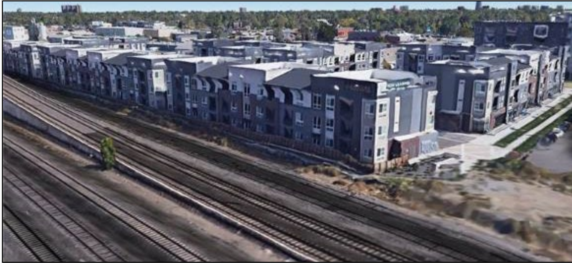
Photo 4-1. Encore Evans Station Apartment Complex
