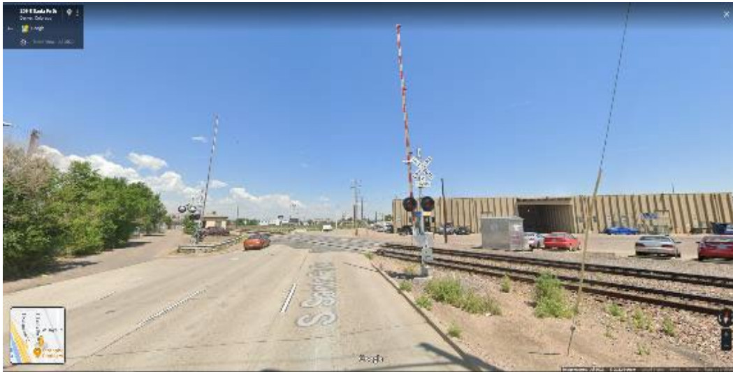
Photo C-3. South Santa Fe Drive Crossing
