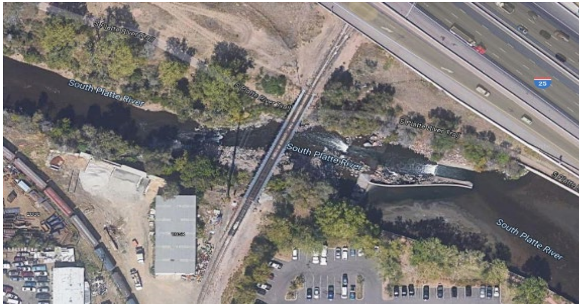
Photo 4-3. Railroad Track Crossing over South Platte River
