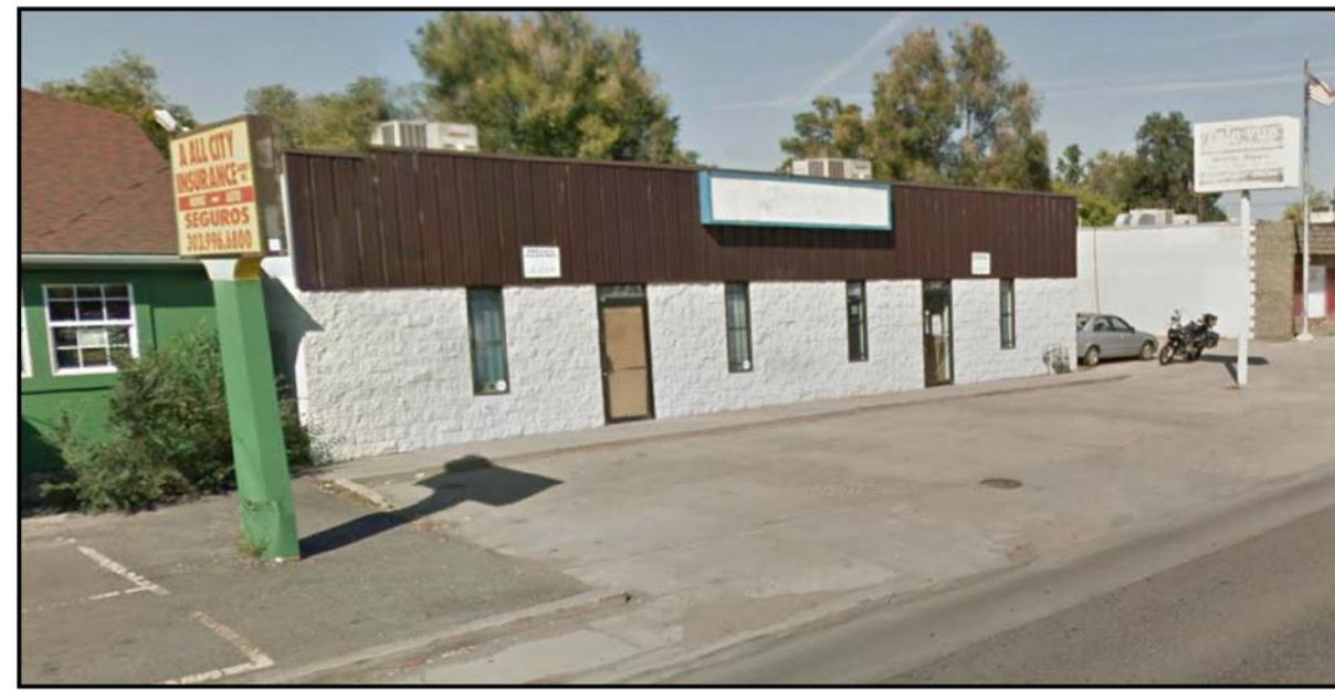
WEST SIDE (STA 31+88)
