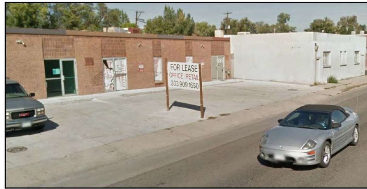
WEST SIDE (STA 27+50)
