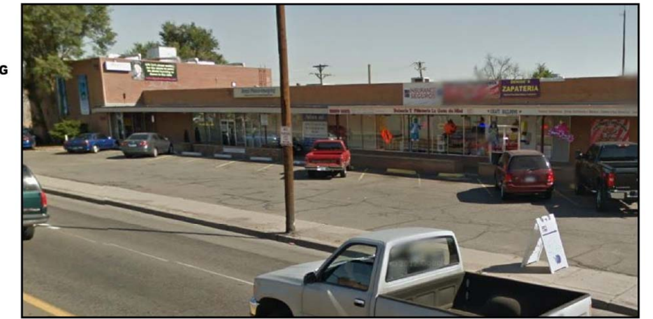
EAST SIDE (STA 27+50)
