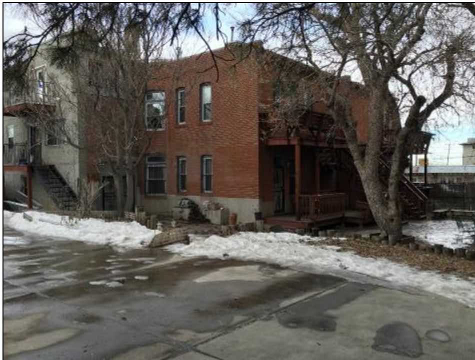
Figure 2. 1940-1946 West 33 rd Ave, rear of “carriage house” and apartment building
