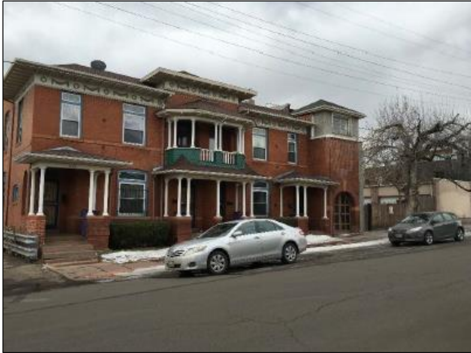
Figure 1. 1940-1946 West 33 rd Ave, apartment building and attached “carriage house”
