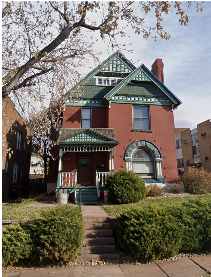
Photo of west facade of 1272 Columbine Street
