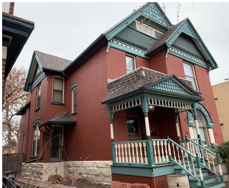
Photo of north and west facades of 1272 Columbine Street (Scott Crotzer, 2020)
