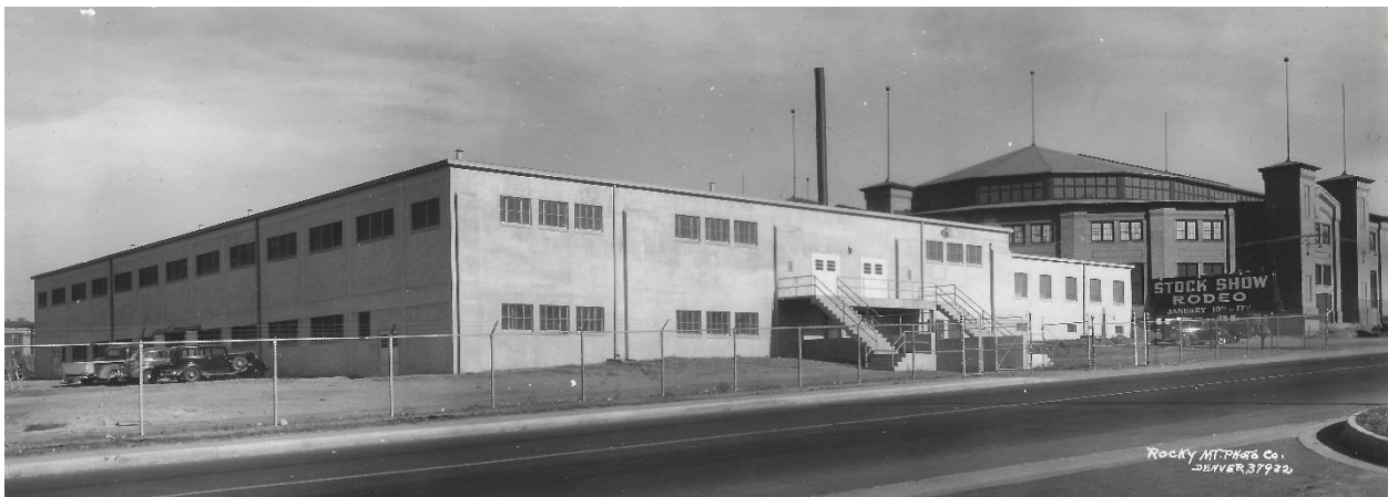
Figure 33. The 1942 WPA-built show barn, which sat on the west side of the Stadium Arena. It was demolished in 1990. Photograph taken approximate 1943. Courtesy NWC archives, February 9, 2016.
