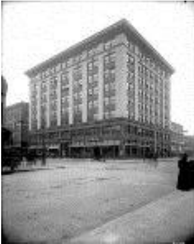
Figure 47. The Symes Building, Hunt and Hunt, 1906. At 16 th Street and Champa Street, Denver, This was the first steel frame building constructed in the city. Source: http://digital.denverlibrary.org/cdm/ref/collection/p15330coll22/id/18946 . Denver Public Library Digital Photograph Collection. Accessed January 20, 2016.
