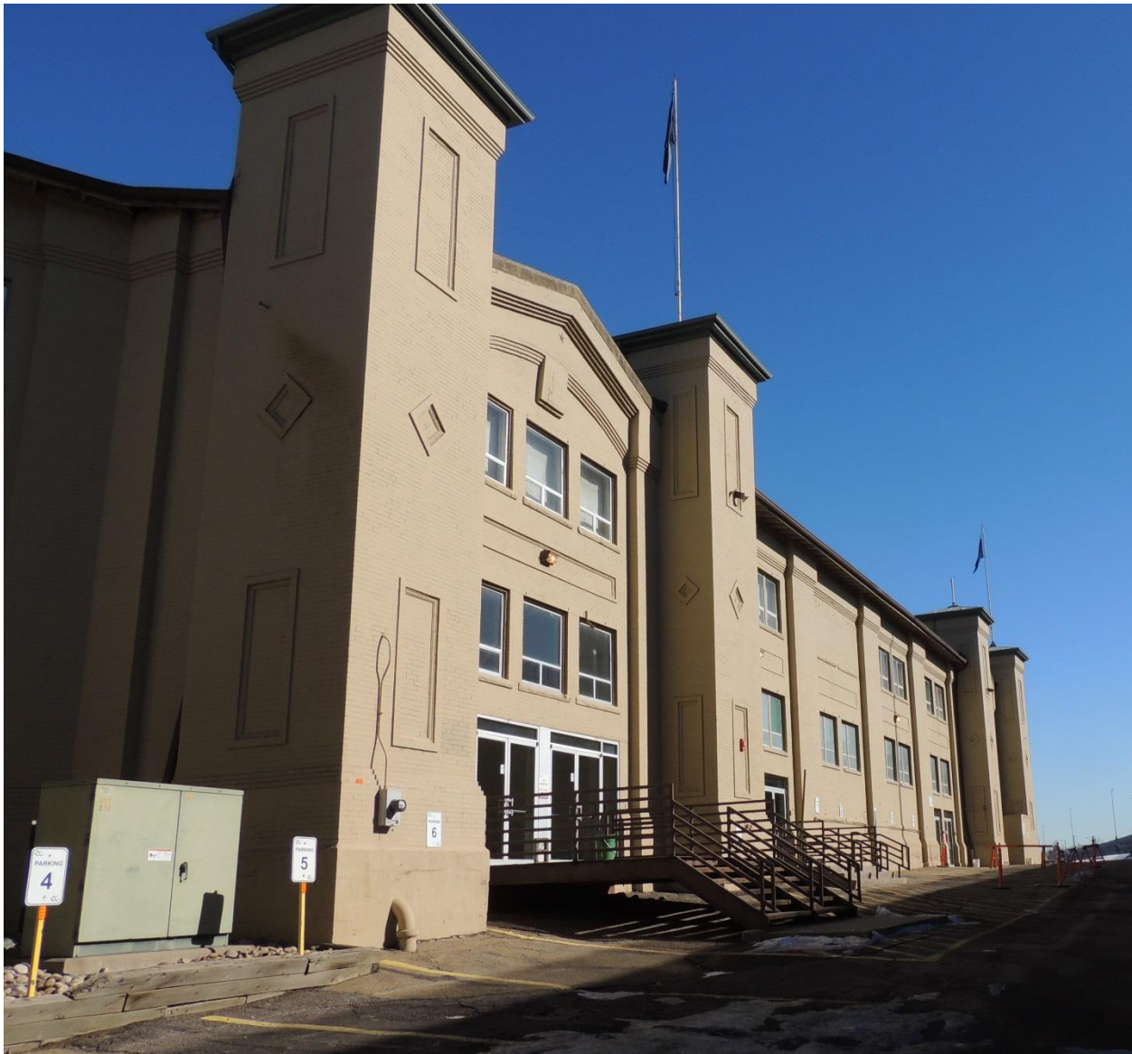
Figure 6. South side of the Stadium Arena, showing the relationship between the entry bays and the bays in between. Facing east-northeast. Photographed February 9, 2016, Dianna Litvak.
