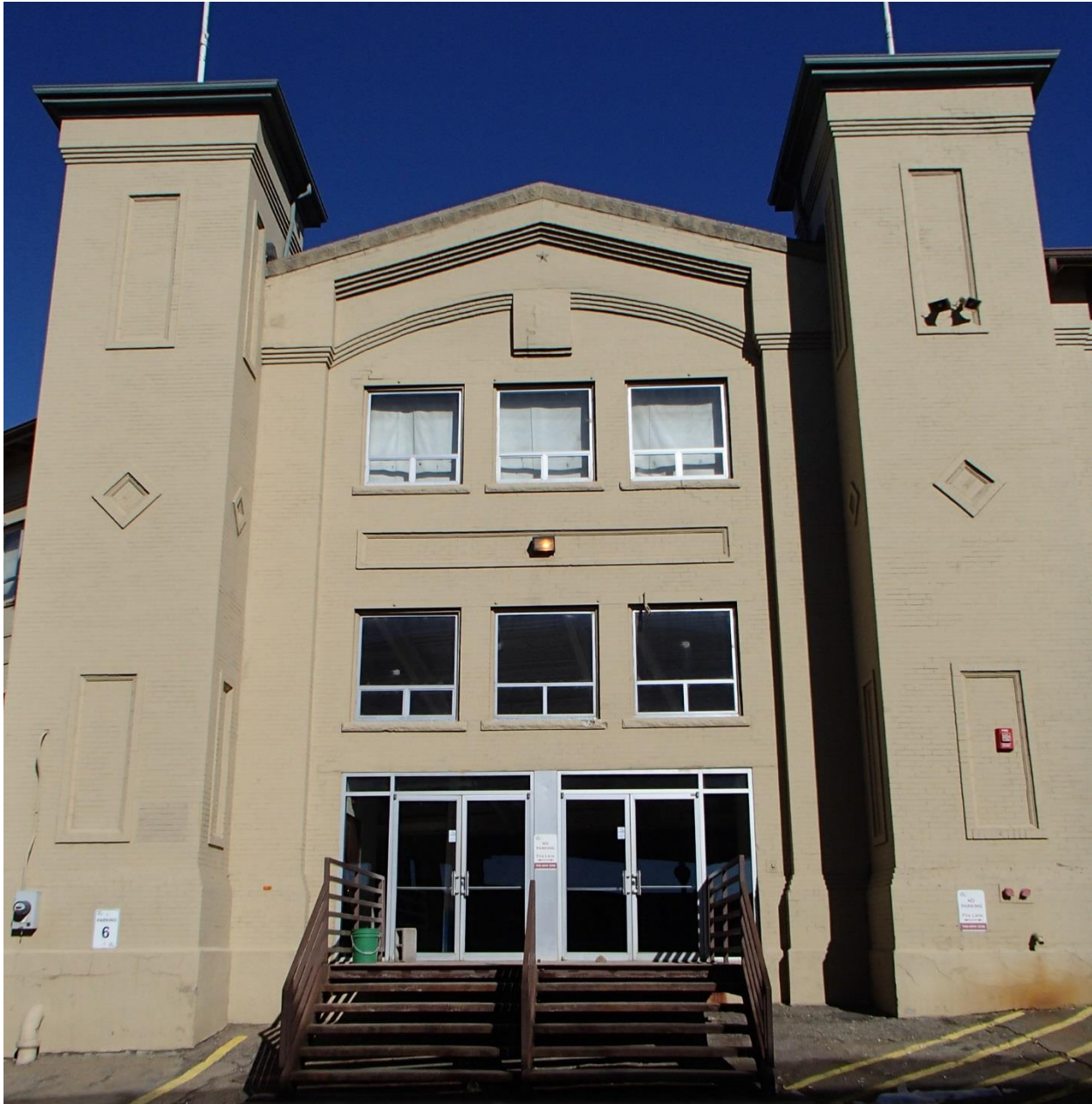
Figure 7. Entrance bay on the south side of the Stadium Arena. Facing north. Photographed February 9, 2016, Kathleen Corbett.
