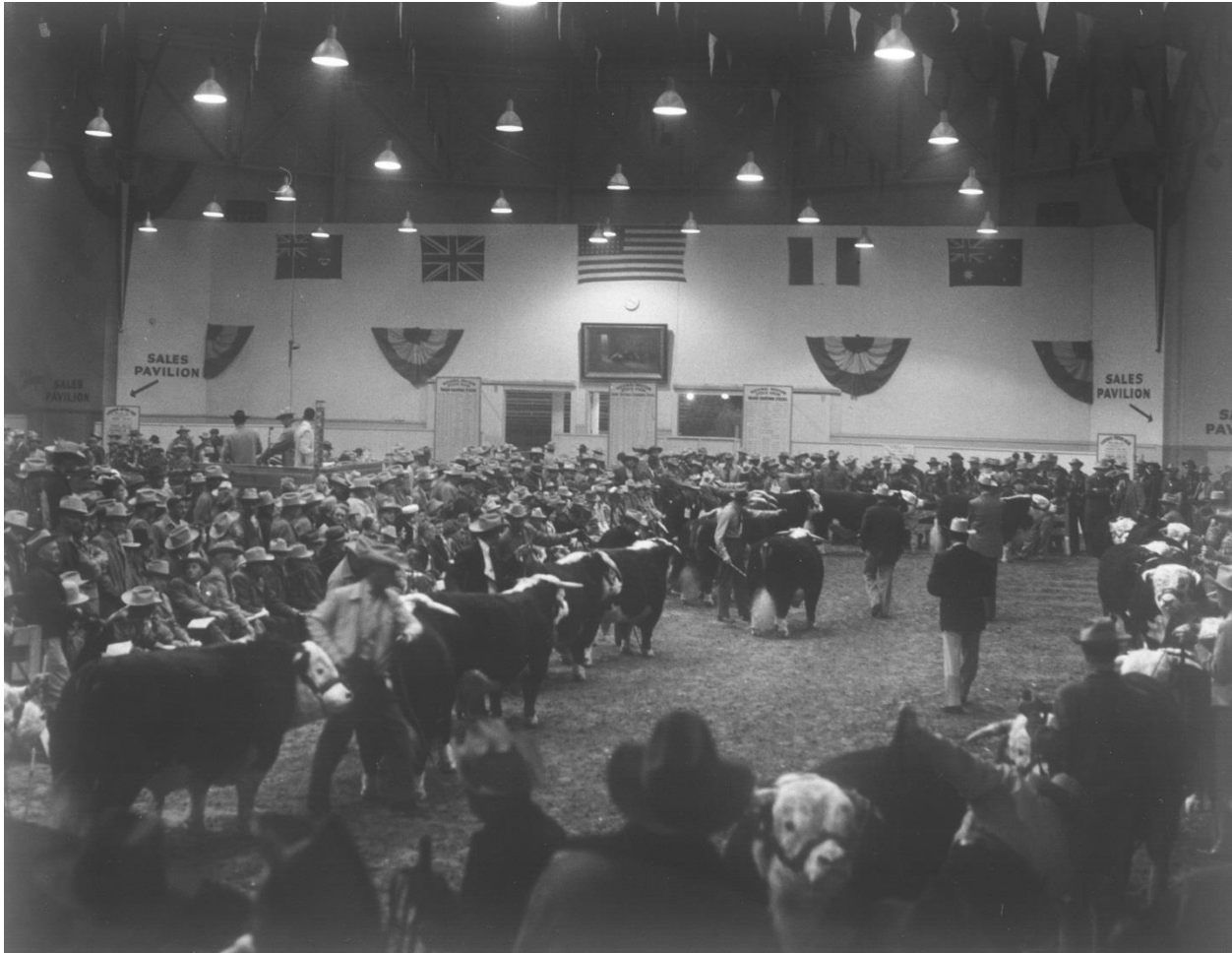
Figure 23. Historic photograph of the 1959 Hereford judging in the Stadium Arena, showing the wall constructed to separate the auction arena from the main arena. Courtesy of the NWC archives, February 9, 2016.
