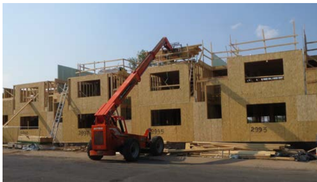
Townhomes east of the subject property
