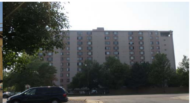
High-rise multi-unit west of the subject property
