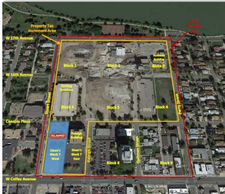
Location of the proposed project within the St. Anthony Urban Redevelopment Area
