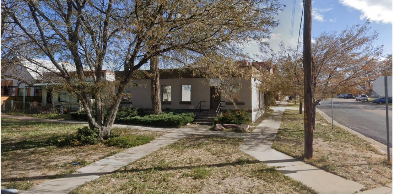
Subject property – from Mariposa Street, looking east.
