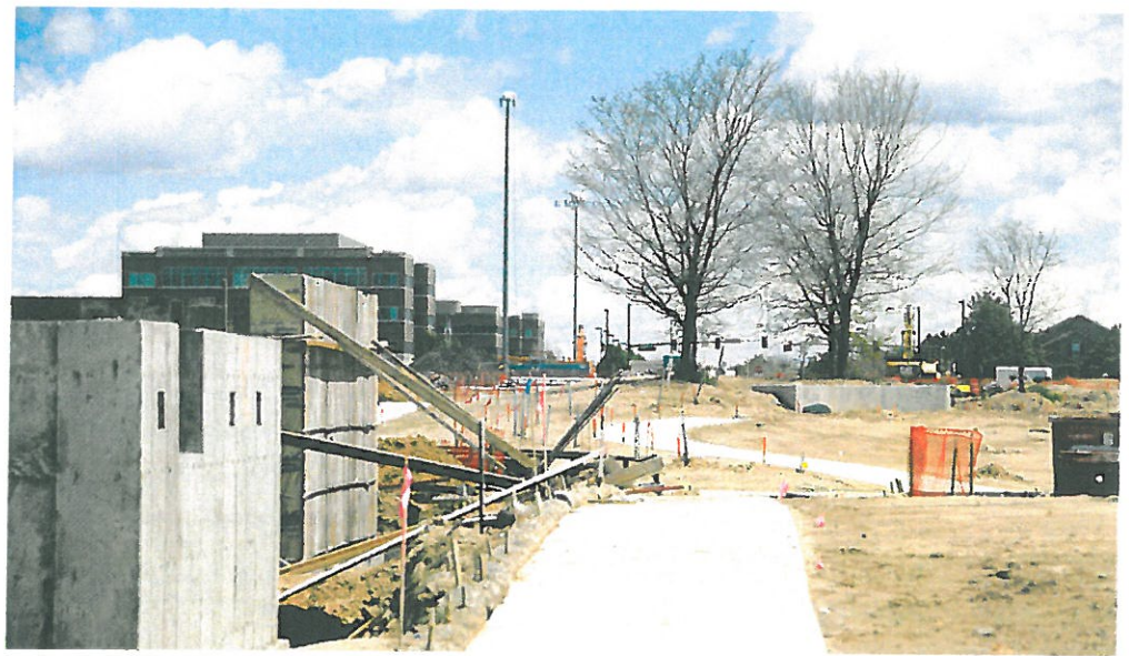
New parks and homes are now under construction at Boulevard One
