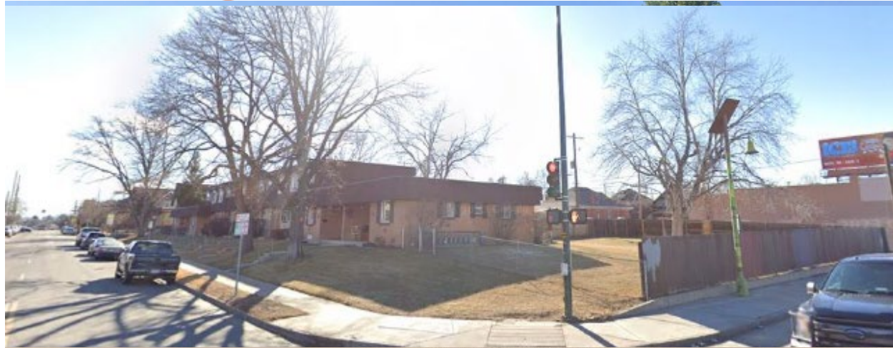
Subject property looking southwest
