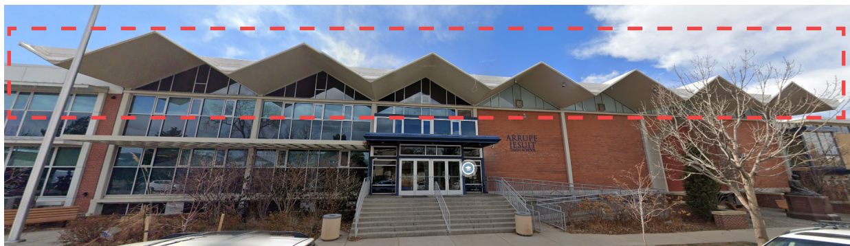
Figure 1-2 Existing folded plate roof (Source: Google Maps)
