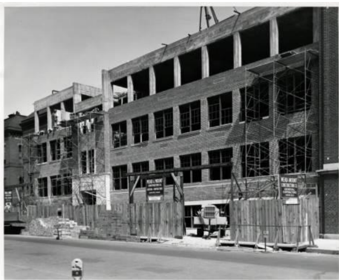
Photo showing construction of the first addition designed by Jamieson. This concrete-frame and brick clad addition was completed in 1947. Photo ca. 1946. Source: Denver Public Library
