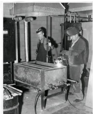
Emily Griffith Opportunity School Welding Class, 1950, Source: Denver Public Library
