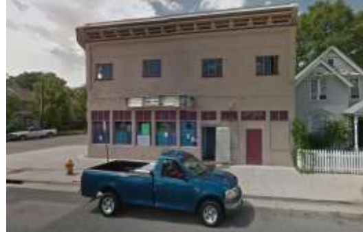
The subject property (image from Google Street View, 2011)
