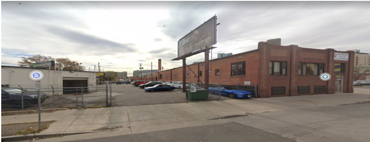
Southeast – from Arapahoe Street (Source: Google Maps)
