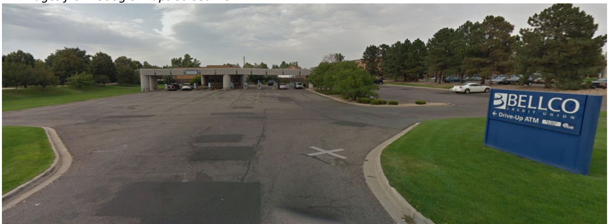
Subject property facing north from E. Mississippi Avenue
