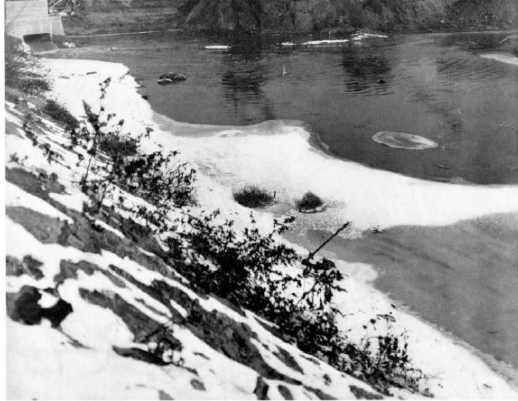
Platte River Flood Protection in Progress Near Globeville
