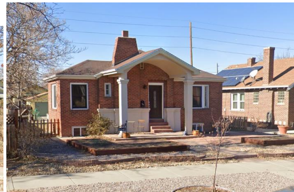
Single Family Residential north of subject property
