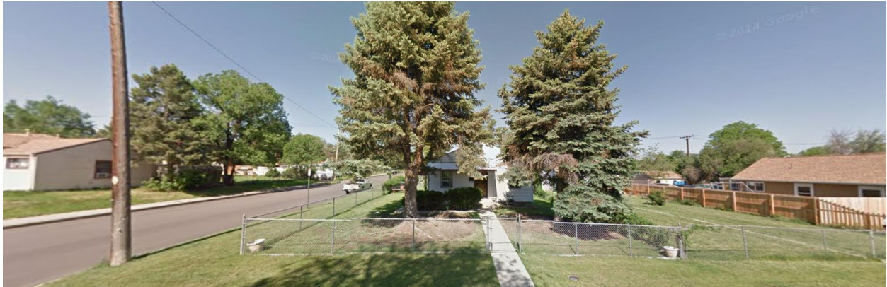
View of the subject property from Irving Street, looking west.
