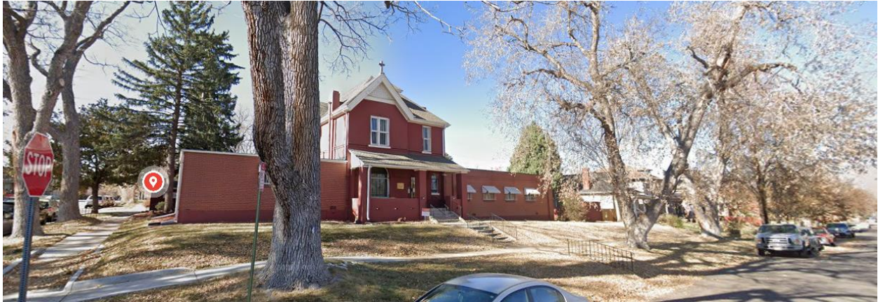
Site, looking west (Source: Google Maps. Note: single-story additions to north and south of building have been removed since this picture was taken)
