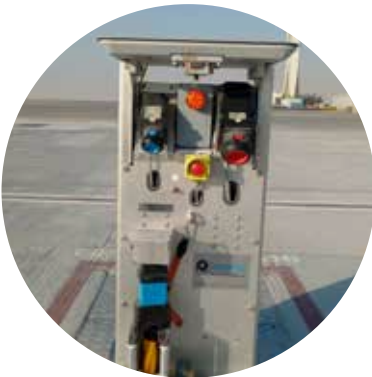
400Hz connector integrated with 400Hz in-ground pit system
