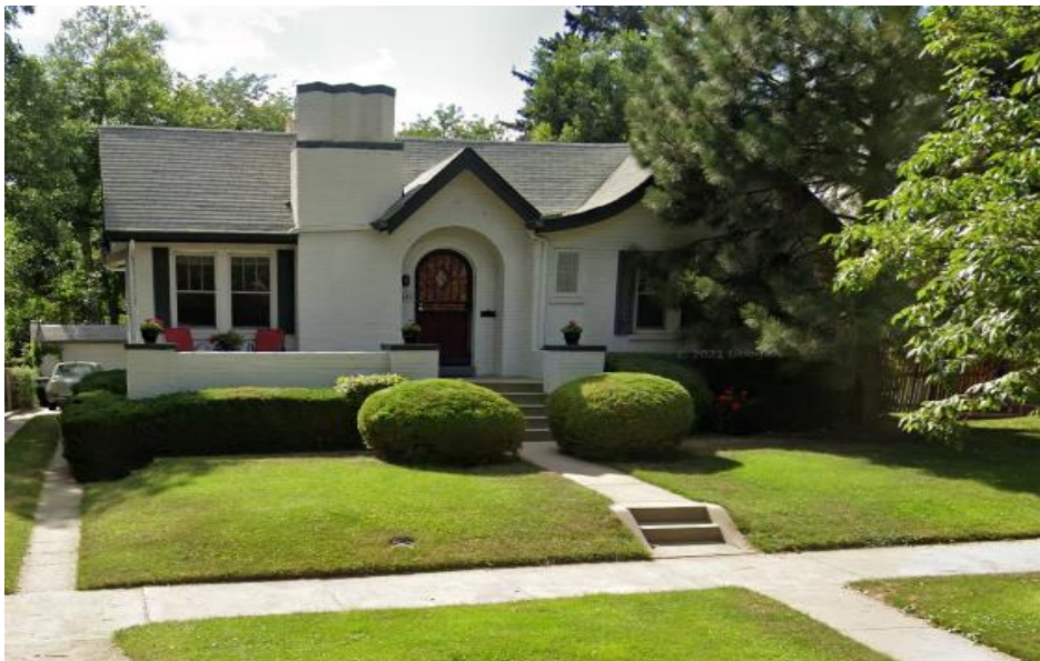
Subject Property - View of 1645 N Grape Street, looking west.
